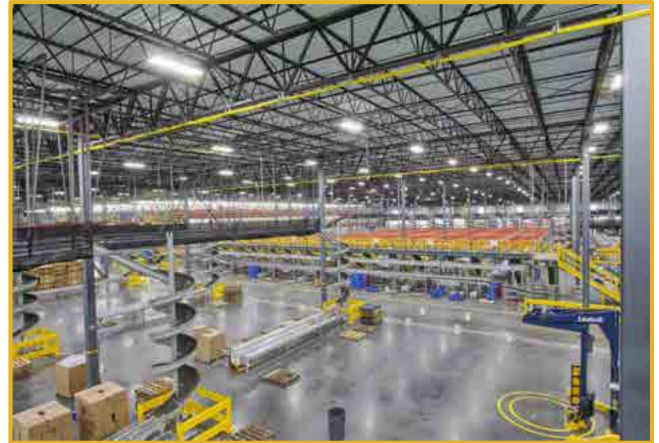
Built-to-Suit Infrastructure Installation (material and handling equipment is owned by tenant)
