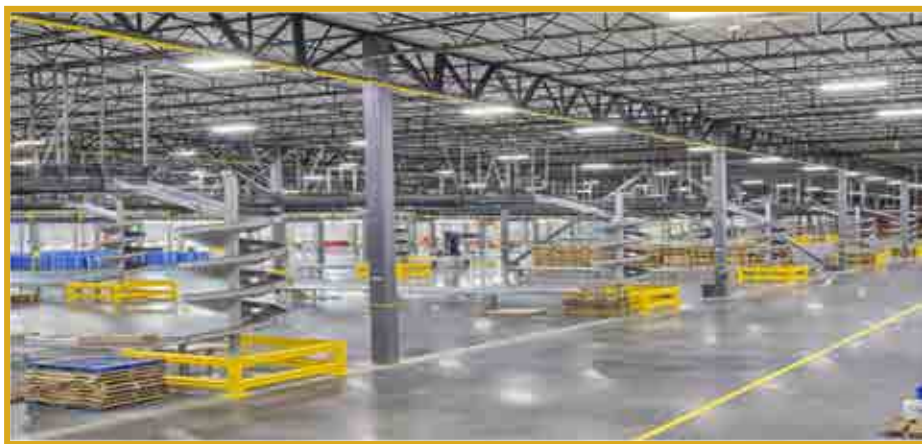
Built-to-Suit Infrastructure Installation (material and handling equipment is owned by tenant)
